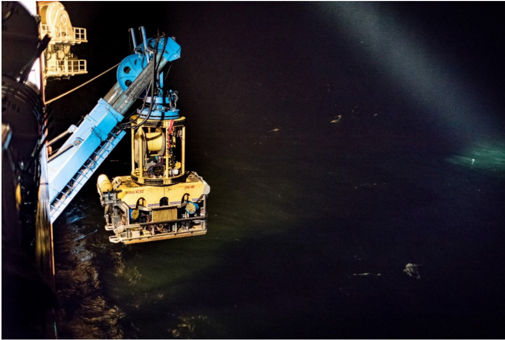
Picture 8. Sea bed studies, laying down ROW in Gulf of Finland
